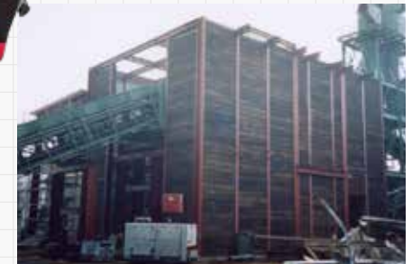
Installation of large shredder
